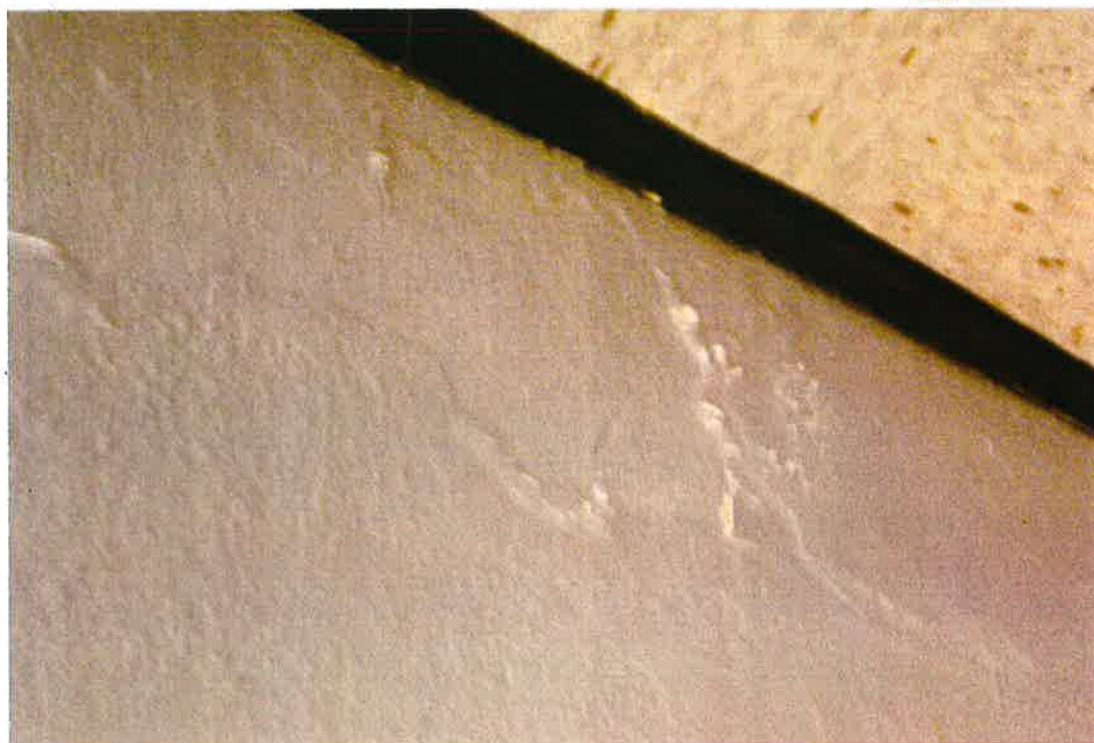
GALLERY Hall moisture from window sills causing walls to crumble North side
