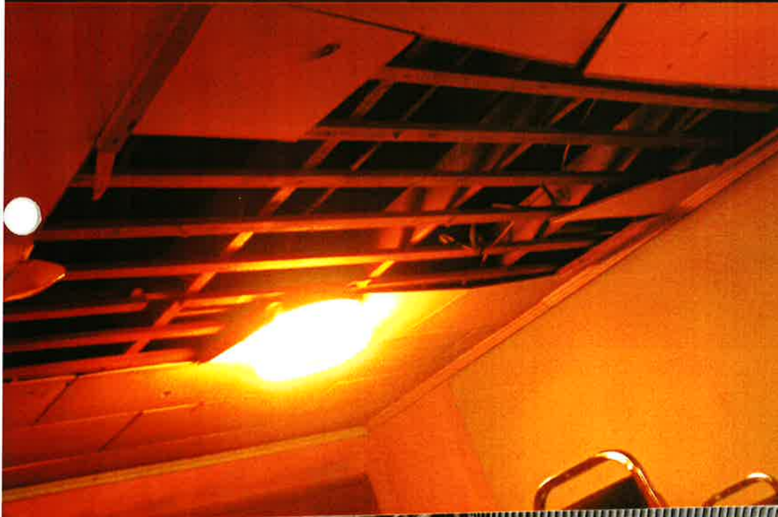
Maintenance Room Ceiling Tile Falling apart
