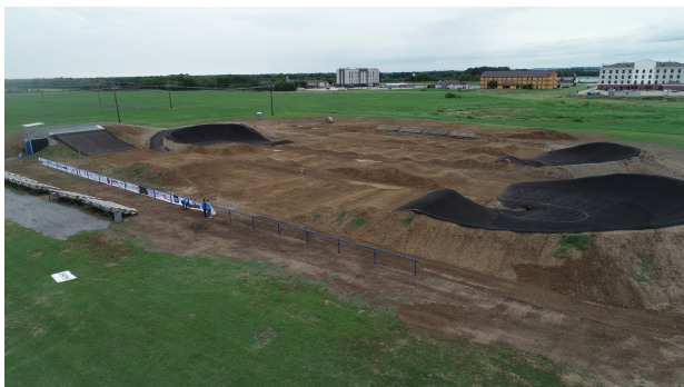
Aerial view of Mayes County BMX
