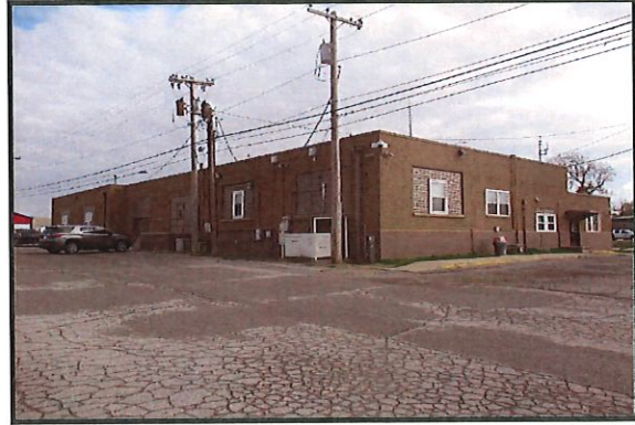
Subject's South and West Elevations
