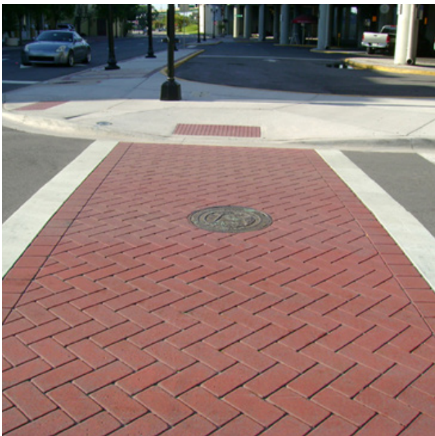
ENHANCED PAVEMENT - CROSSWALK PATTERNED STAMPED CONCRETE
