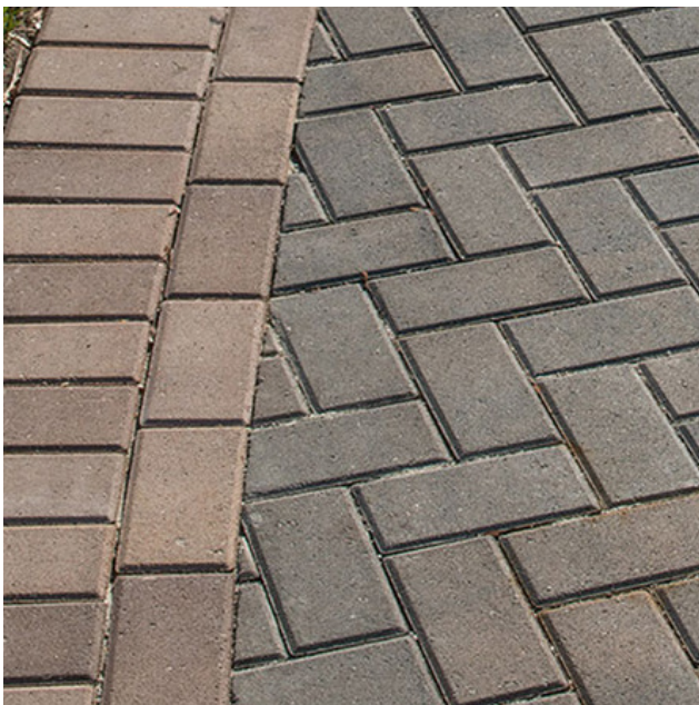
ENHANCED PAVEMENT - SIDEWALK KEYSTONE - HOLLAND PAVER
