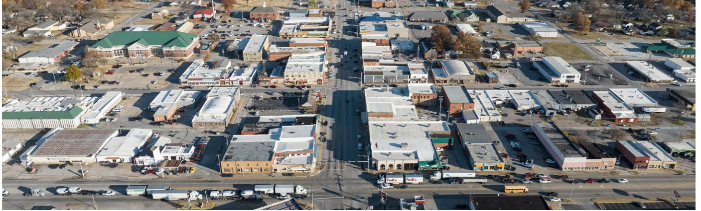
City of Pryor Creek along State Highway 69
