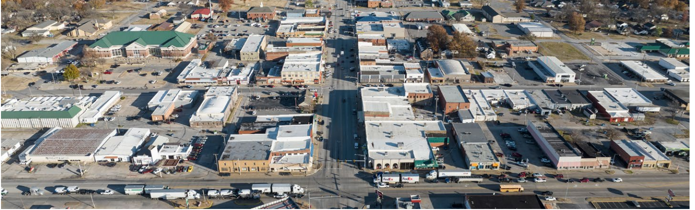
City of Pryor Creek along State Highway 69
