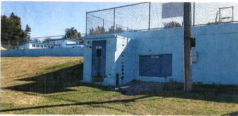
Chemical storage building.
